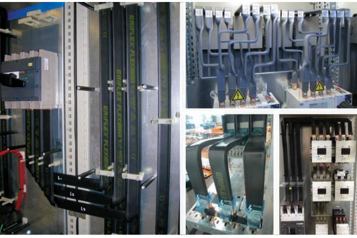
Application pictures: Flexibar directly connected on various devices or rigid bars, with compact connection and from 125 A up to 4500A
