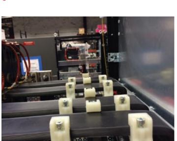
Application pictures: Flexibar fixed/secured with nVent ERIFLEX spacers and clamps.
