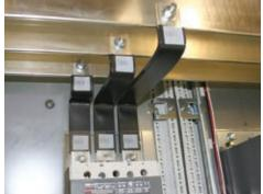
Application pictures: Flexibar directly connected on MCCB's front access connection.
